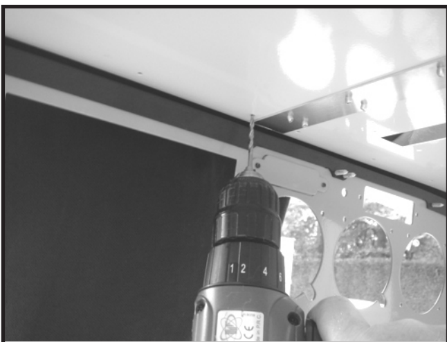
45. From the inside, drill a hole through the glareshield in the middle through an existing white sheet hole, while holding the cabinet and glareshield in the same position.
